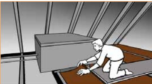
**STEP 4** - Where the depth of previously installed insulation has reached the tops of the joists, extra heat saving is gained by 'cross layering' (at right angles to joists) with 150mm or 170mm Space Loft Roll (or 200mm for even higher energy savings).
