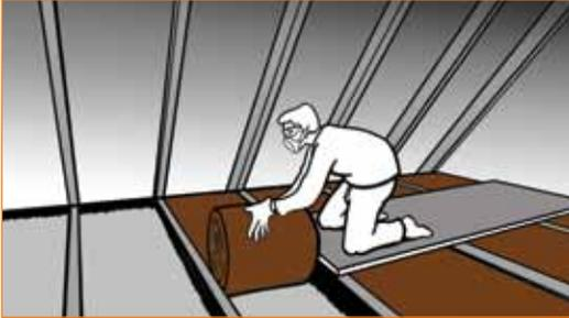
**STEP 2** - When space along the joists is filled, the end of the roll can be turned back to start an extra layer of insulation or may be cut to size.
